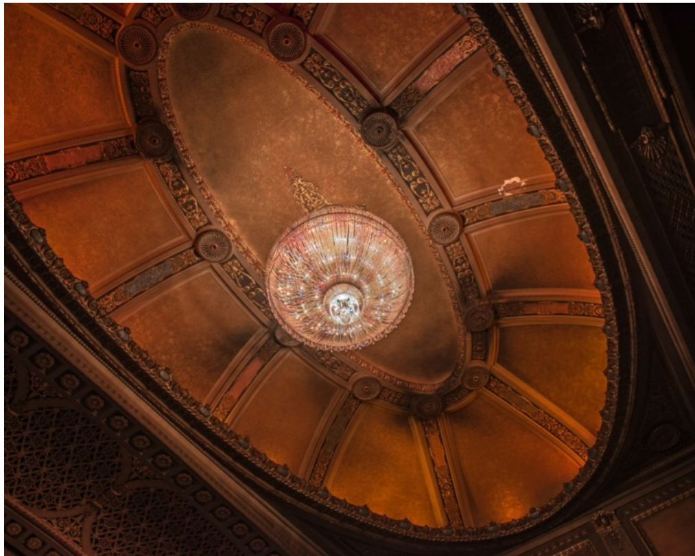
This is a shot showing some of the lost art of ceiling decoration. Also shown is the main chandelier.
